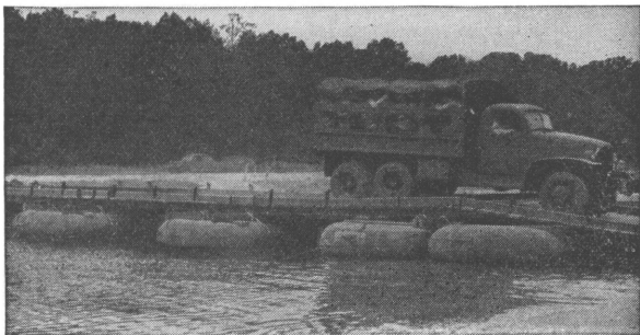
FIGURE 122.—Pneumatic bridge.
