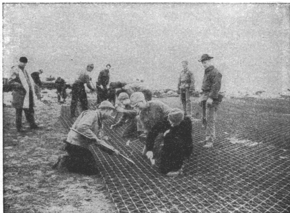
FIGURE 138.—Laying Irving grid steel runway.
