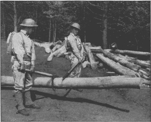
FIGURE 40.—Using the peavy to carry heavy timber.
