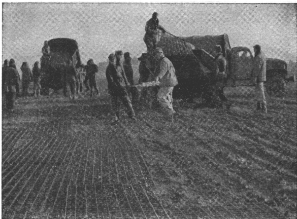
FIGURE 139.—Laying bar-and-rod type steel runway.
