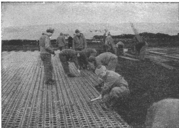
FIGURE 137.—Laying pierced plank steel runway.
