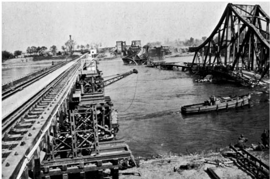
Above: The Wesel rail bridge built by American Engineers, Seabees and Transportation personnel was situated just a few yards from the downstream side of the road bridge. By V-E Day, the eastbound freight over this one bridge had amounted to 273,141 tons. Other American rail bridges were the President Roosevelt Bridge at Mainz (see page 40) and the Victory Bridge at Duisburg.
