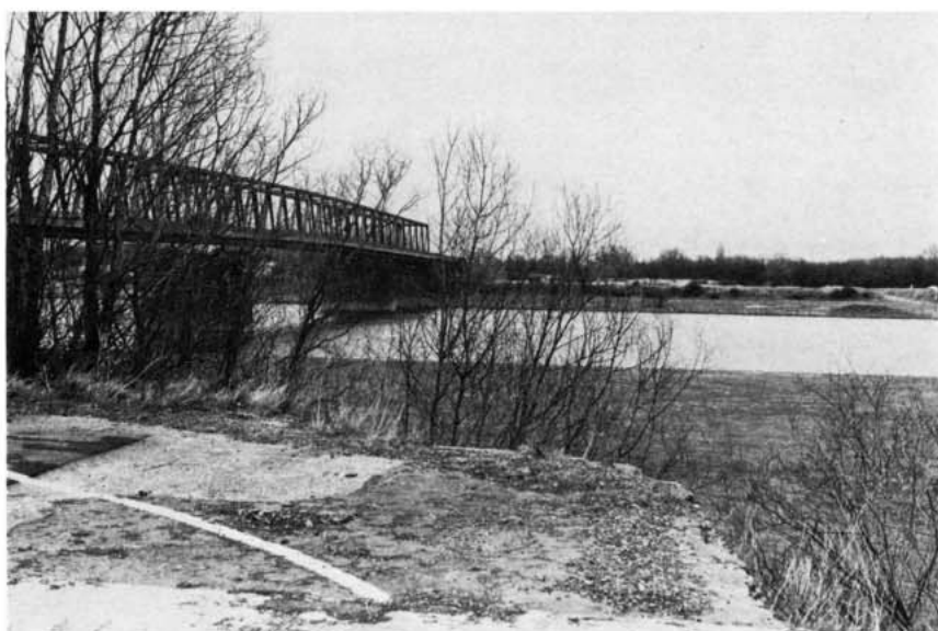
Above: The semi-permanent road bridge at Wesel built by the 1146th Combat Engineer Group beside the demolished road bridge photographed by Pfc N. Sperry of the Signal Corps. Below: The bridge was later replaced by the all-weather Montgomery Bridge. Today, the old approach road is still visible beside the rebuilt permanent bridge.
