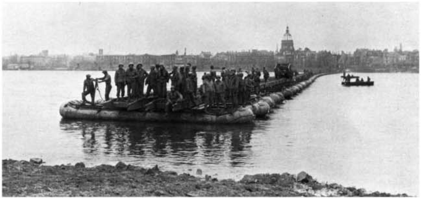
Above: Third Army engineers of the 80th Division claimed that the 'Sunday Punch' ponton treadway at Mainz, was the longest assault bridge across the Rhine at 1,865ft (US Signal Corps). Below: The restored Cristuskirche is a prominent landmark today.
