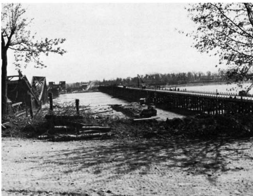
Above: The semi-permanent road bridge at Wesel built by the 1146th Combat Engineer Group beside the demolished road bridge photographed by Pfc N. Sperry of the Signal Corps. Below: The bridge was later replaced by the all-weather Montgomery Bridge. Today, the old approach road is still visible beside the rebuilt permanent bridge.
