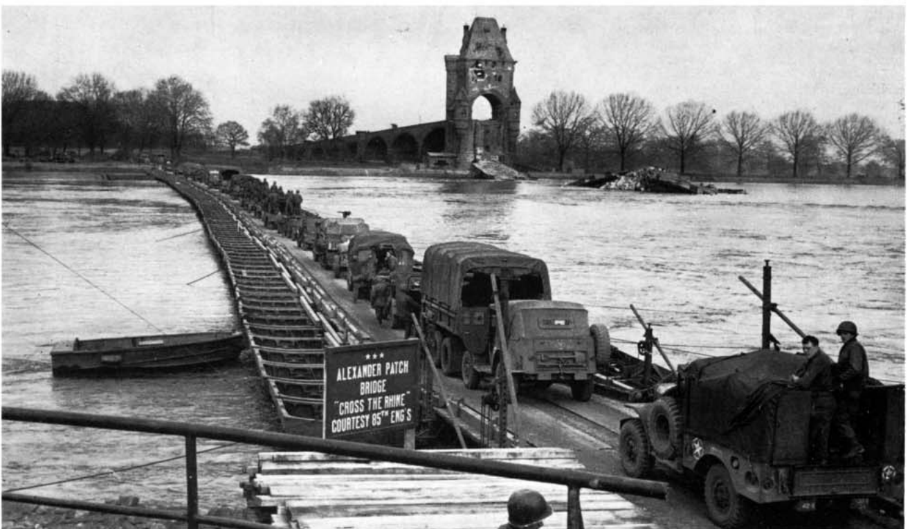
Top and above: The 63rd Division crosses the 1,164ft bridge built by the 1014th and 1019th Engineer Treadway Companies at Hamm. Photographer 2nd Lieutenant J. Harris, US Signal Corps.
