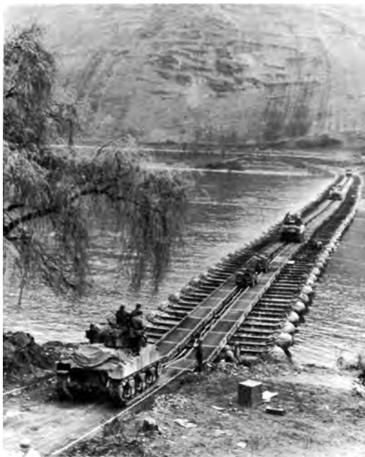
M2 TREADWAY BRIDGE on the Rhine at Boppard.
