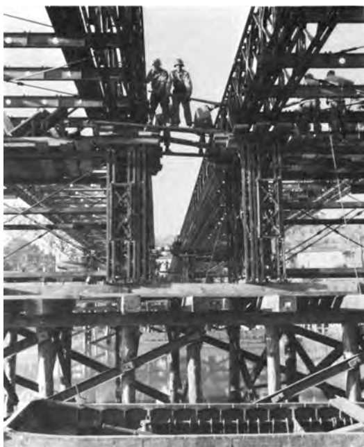
BAILEY BRIDGE CONSTRUCTION over the Arno near Florence.
