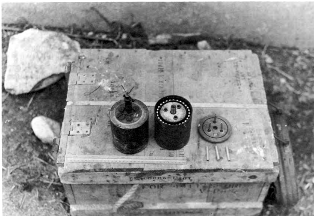
GERMAN S-MINE. The activated canister burst from the earth and fired over 300 steel pellets in all directions.
