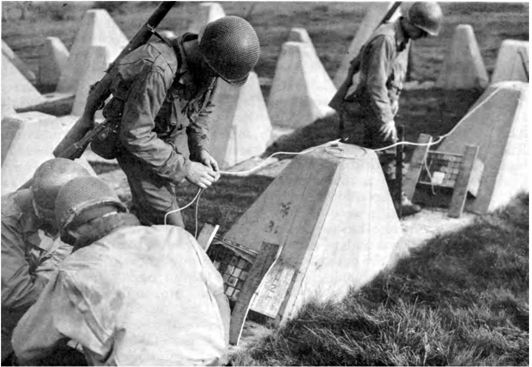
MEN OF THE 23D ARMORED ENGINEER BATTALION RIG CHARGES to demolish dragon's teeth in the Siegfried Line.
