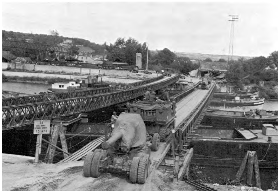
FRENCH BARGES SUPPORT BAILEY BRIDGING OVER THE SEINE AT MANTES
