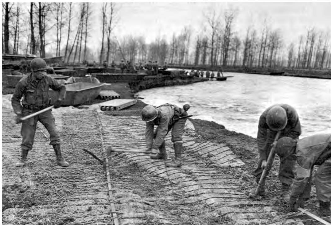
ENGINEERS EMPLACE MATS TO STABILIZE THE BANKS OF THE FLOODED ROER
