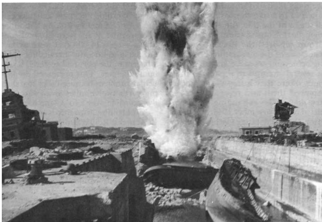
BLAST REMOVES BLOCKAGE FROM THE MOUTH OF THE LOCKS AT ST. MALO
