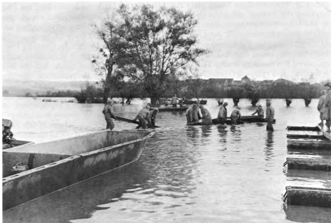
TROOPS FLOAT FOOTBRIDGE SECTIONS INTO PLACE on the flooded Moselle River in the 90th Division area.
