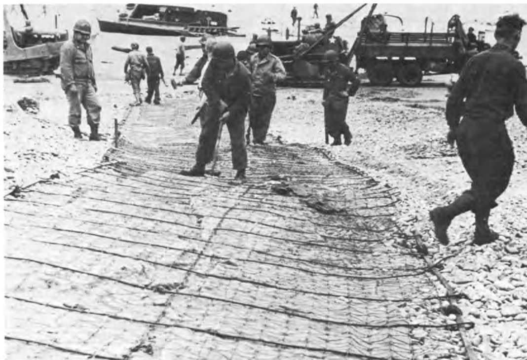
ENGINEERS ANCHOR REINFORCED TRACK for vehicles coming ashore at Omaha.
