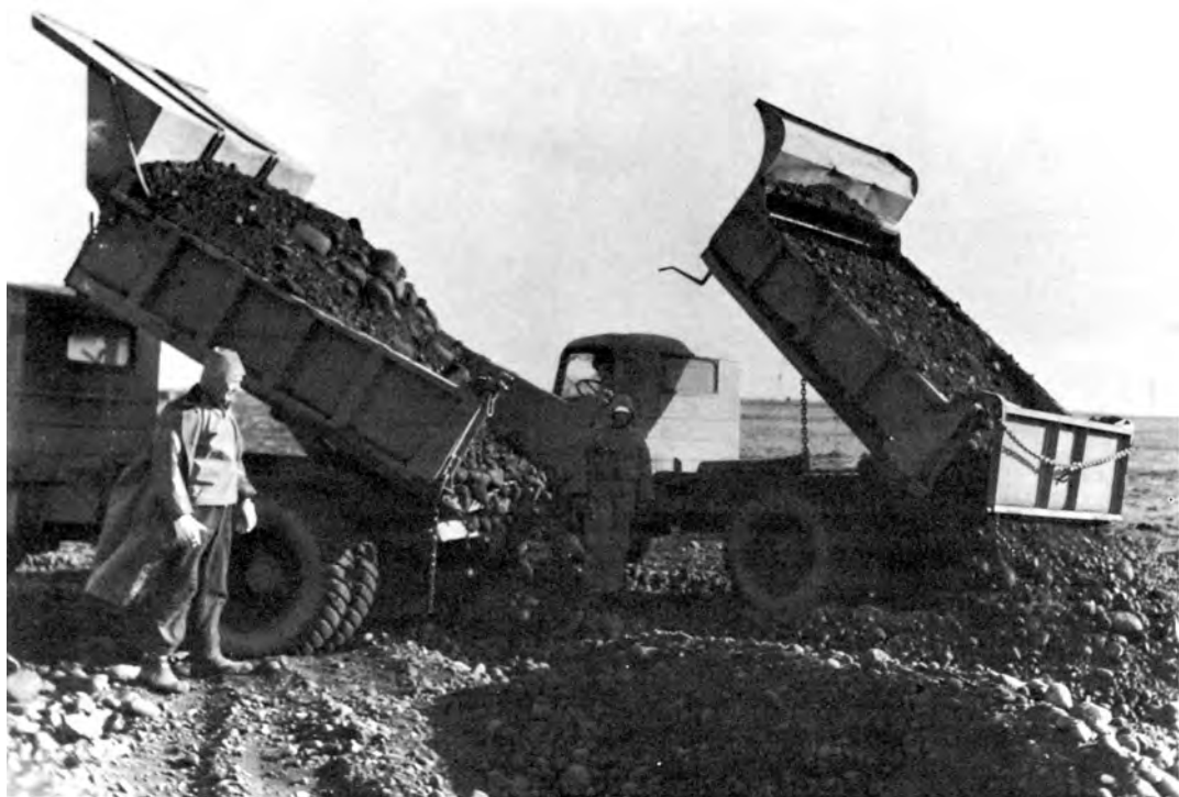
ENGINEER TROOPS DUMPING FILL AT MEEKS FIELD, KEFLAVIK
