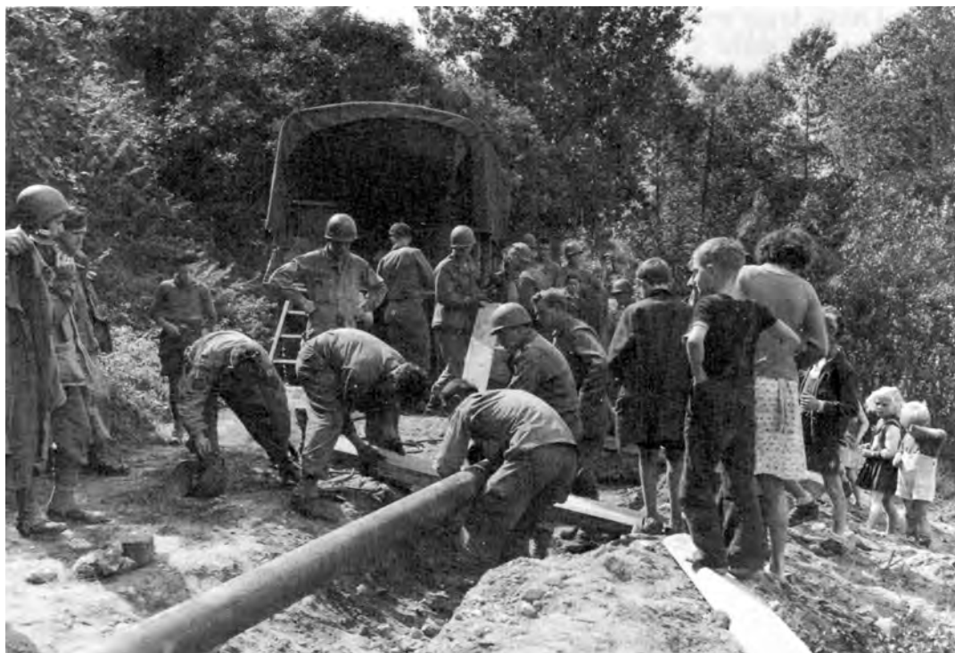
FRENCH CHILDREN WATCH THE 982D ENGINEER MAINTENANCE COMPANY WELD SIX-INCH PIPELINE
