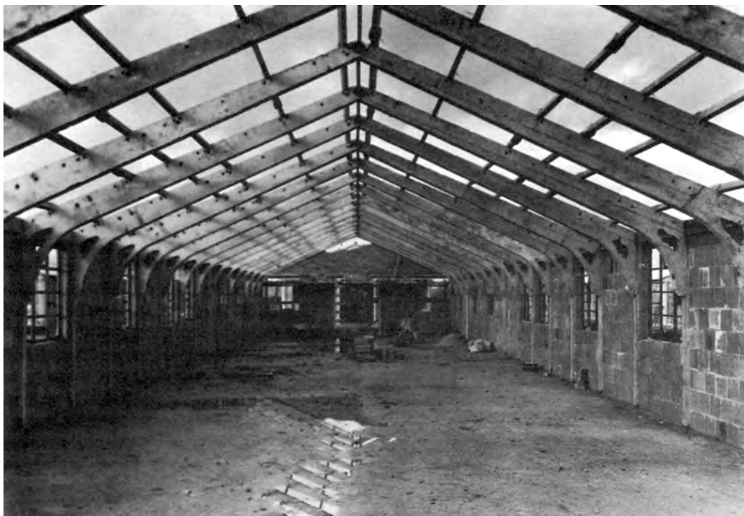
HOSPITAL CONSTRUCTION EMPLOYING PREFABRICATED CONCRETE ROOF TRUSSES
