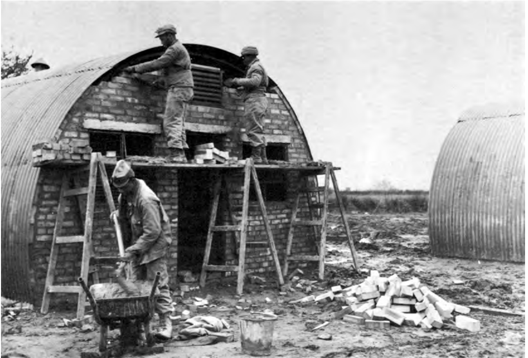
MEN OF THE 829TH ENGINEER AVIATION BATTALION ERECT NISSEN HUTTING
