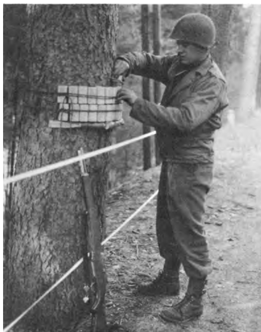
PLACING CHARGES TO DROP TREES across roadways.
