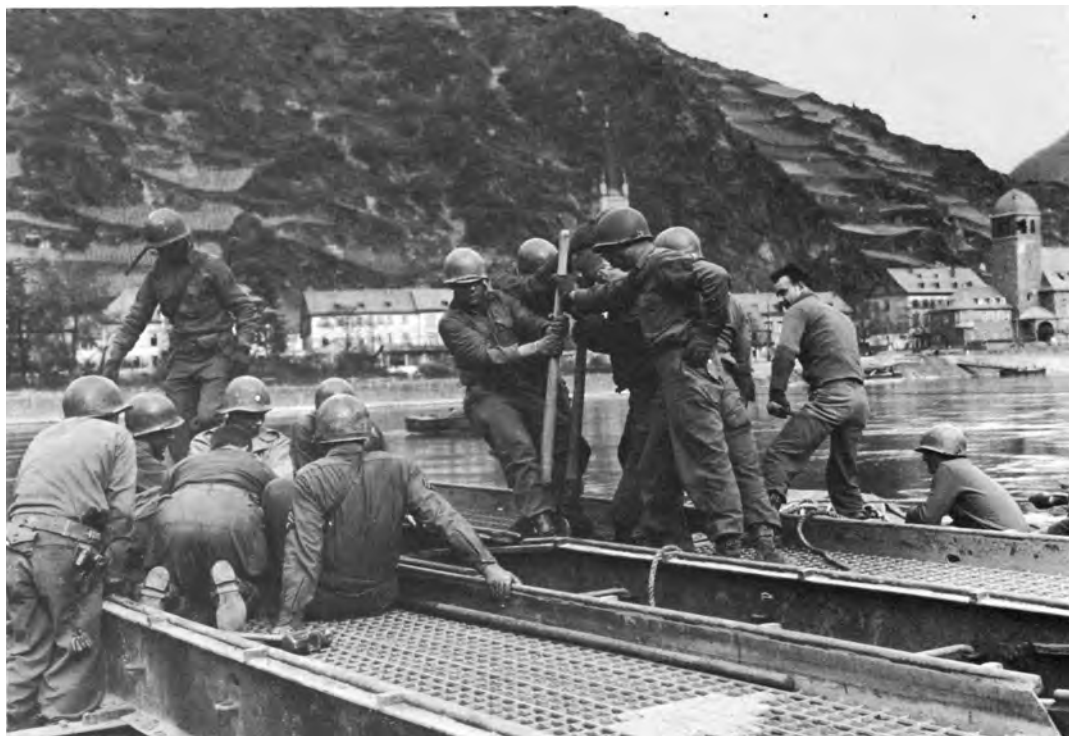
MEN CONNECT BRIDGE SECTIONS NEAR ST. GOAR
