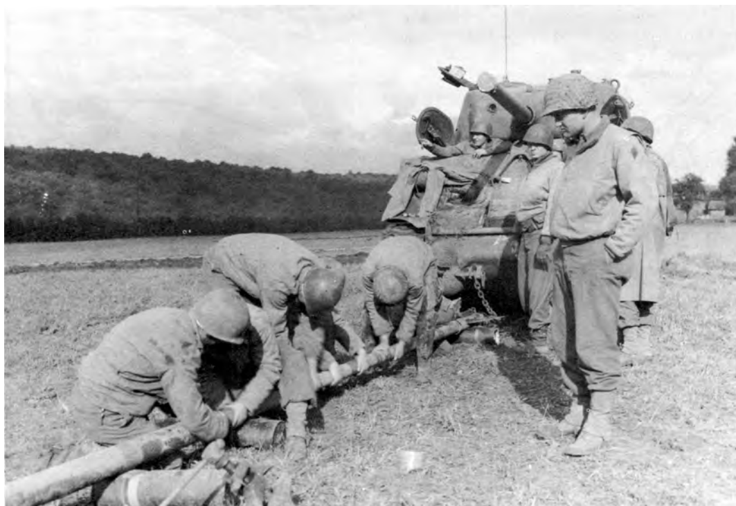
ENGINEERS ASSEMBLE AN EXPLOSIVE-LADEN "SNAKE" to clear a path in a minefield.
