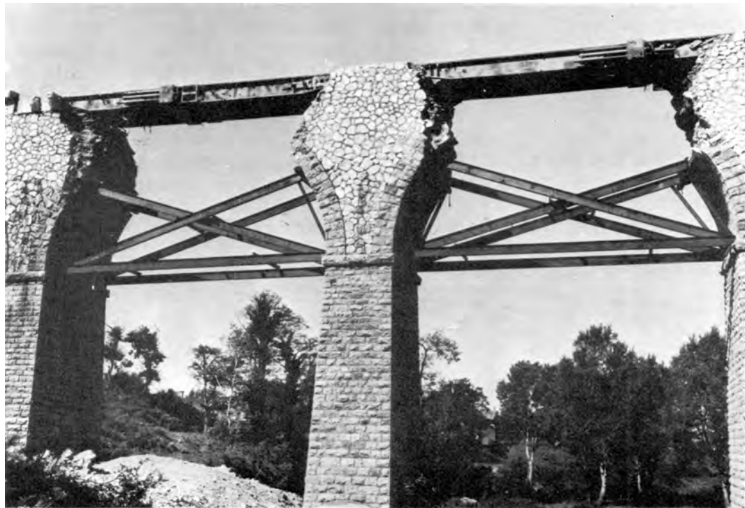
THE AIX BRIDGE, WHICH USED THE CARRIAGE OF A GERMAN RAILWAY GUN
