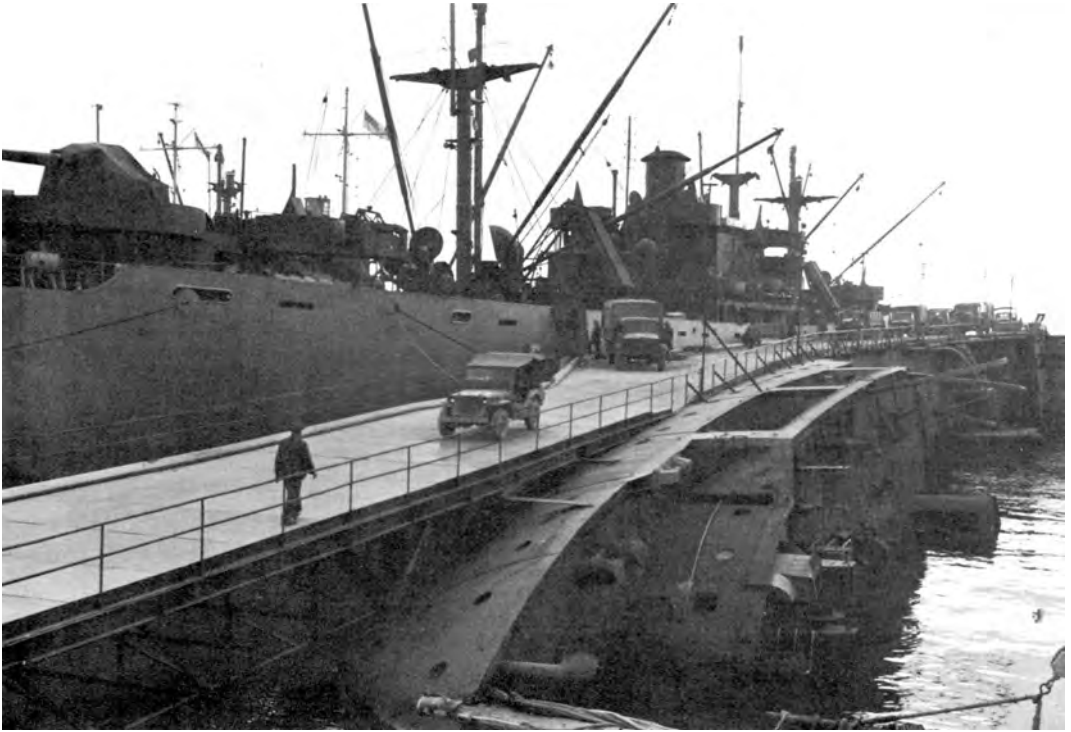
DECKING PLACED OVER SUNKEN VESSELS to enable loading in Naples harbor.
