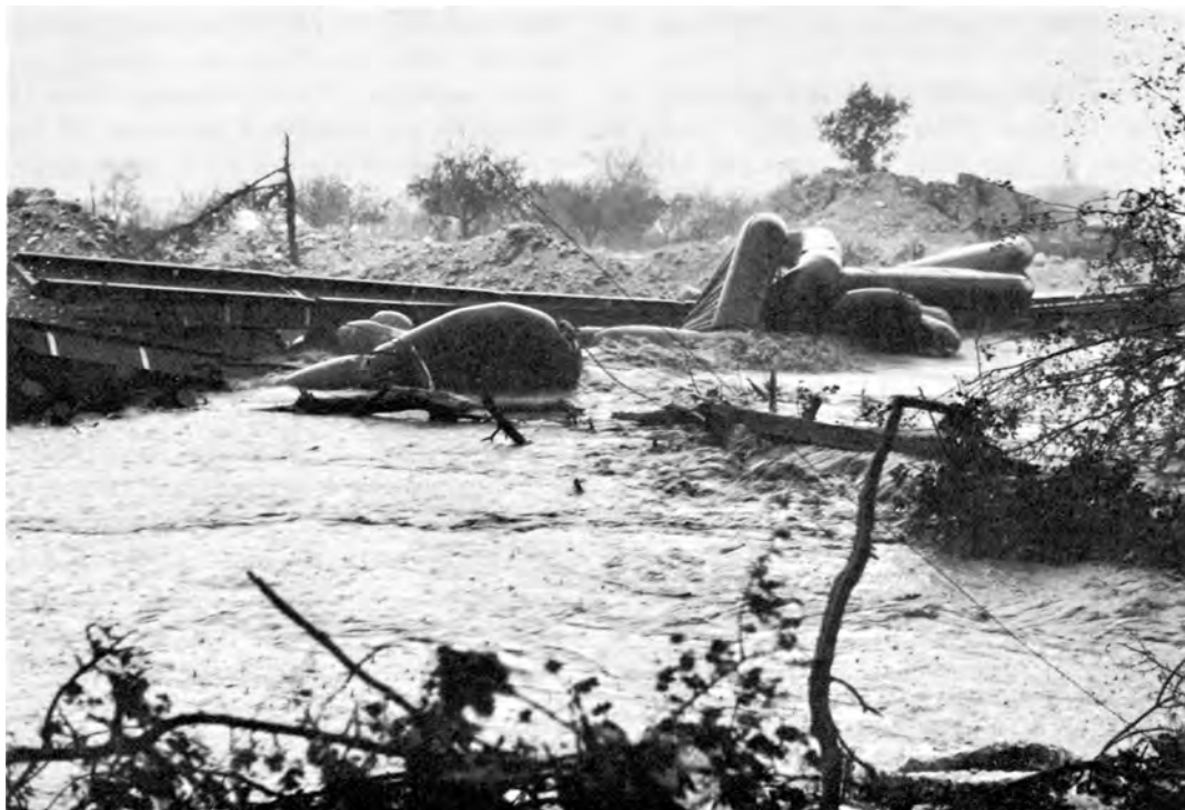
WRECKED M2 FLOATING TREADWAY ON THE VOLTURNO
