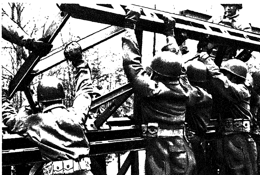
Figure 8-9. Placing outer-truss second-story panel for converting double-single to double-double bridge.
