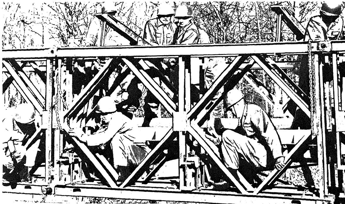
Figure 7-39. Inserting panel of outer truss. Note use of levers and chain slings to lower panel into position.
