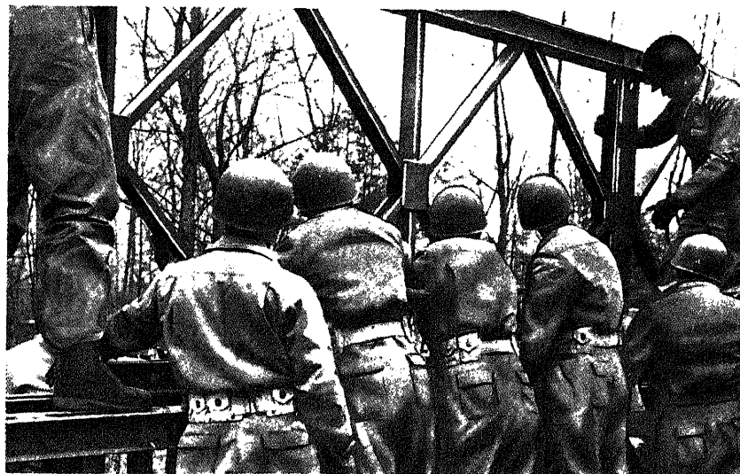
Figure 8-10. Outer second-story panel in position before insertion of panel pins.
