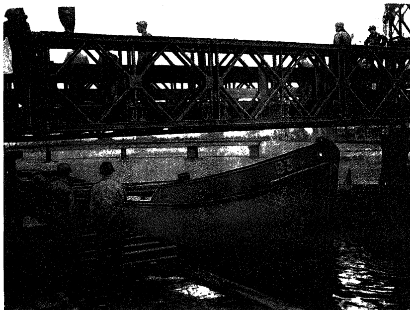
Figure 20-24. Lift span raised for river traffic. Note use of span junction posts.
