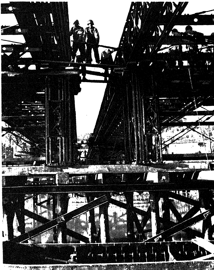
Figure 17-43. Two panel bridges being jacked down onto panel crib piers.
