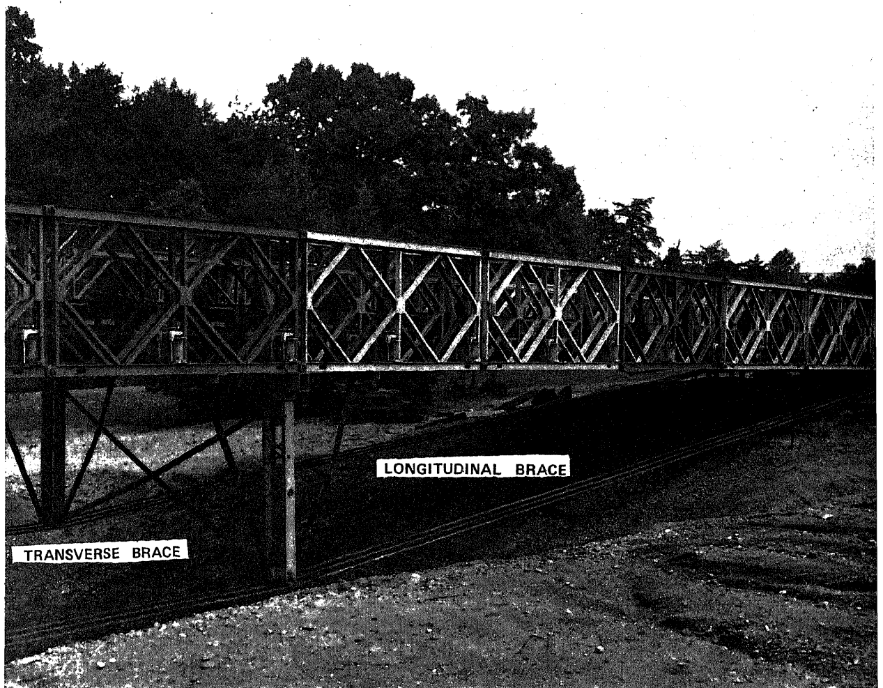
Figure 15-3. Cable reinforcement set vertical posts installed on Bailey bridge.
