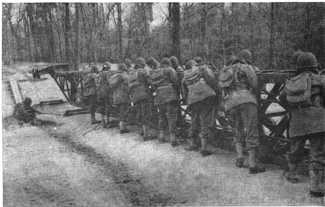
FIGURE 31.—Truss being pushed out on erection rollers.
