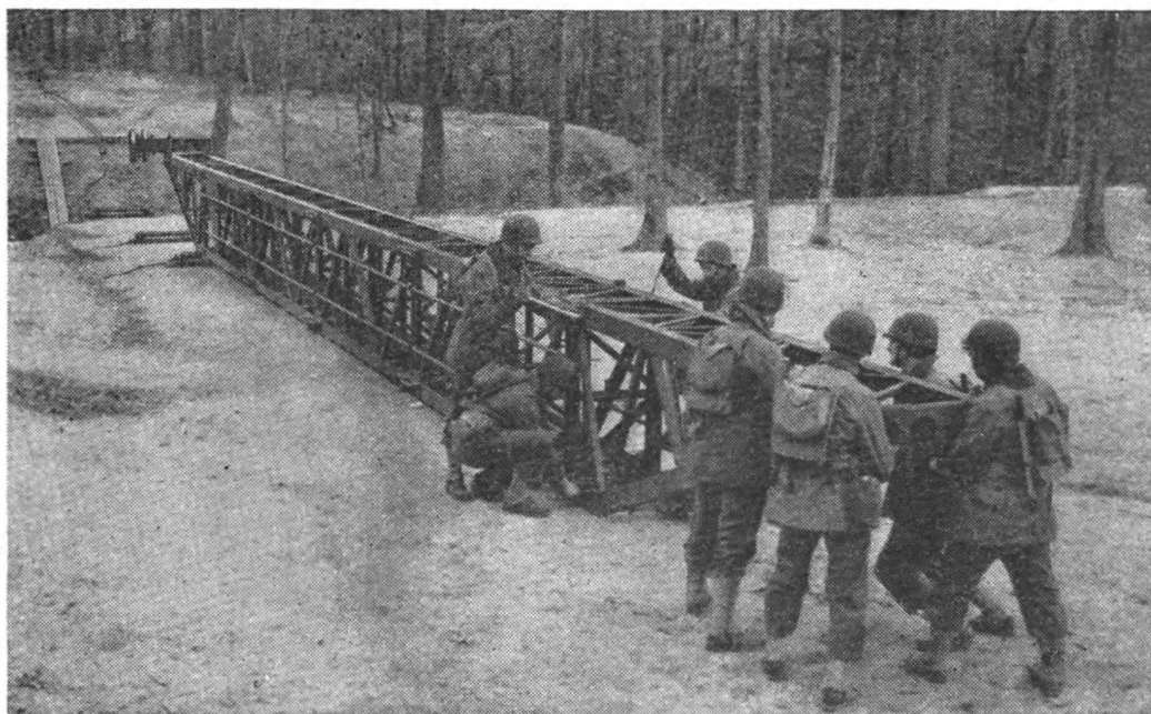
FIGURE 23.—Last section of truss being bolted.
