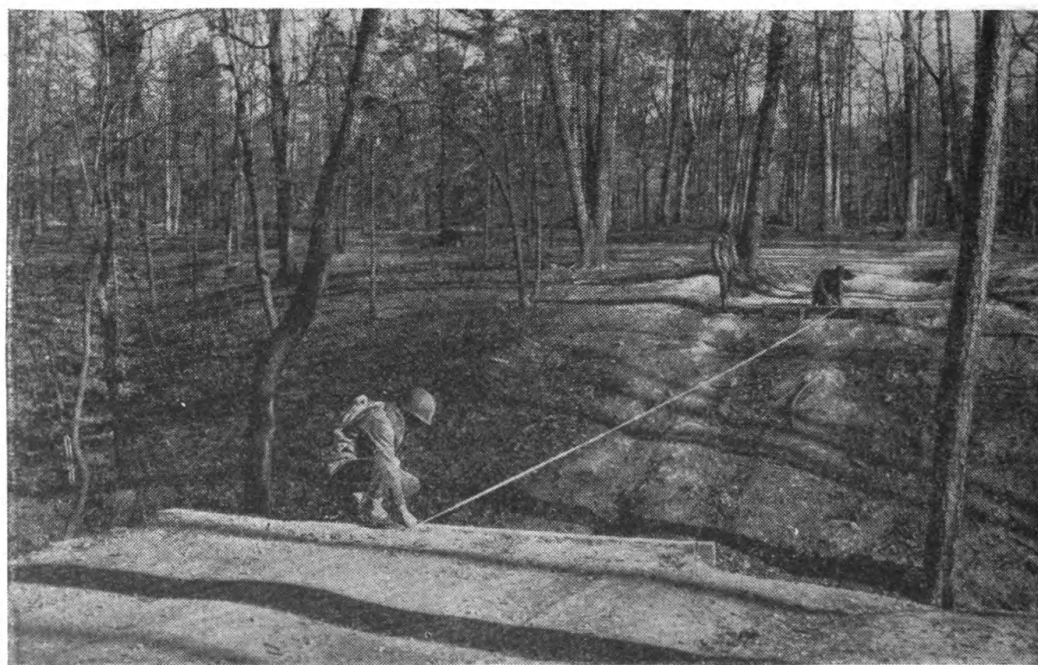
FIGURE 29.—Distance between abutment sills being checked.
