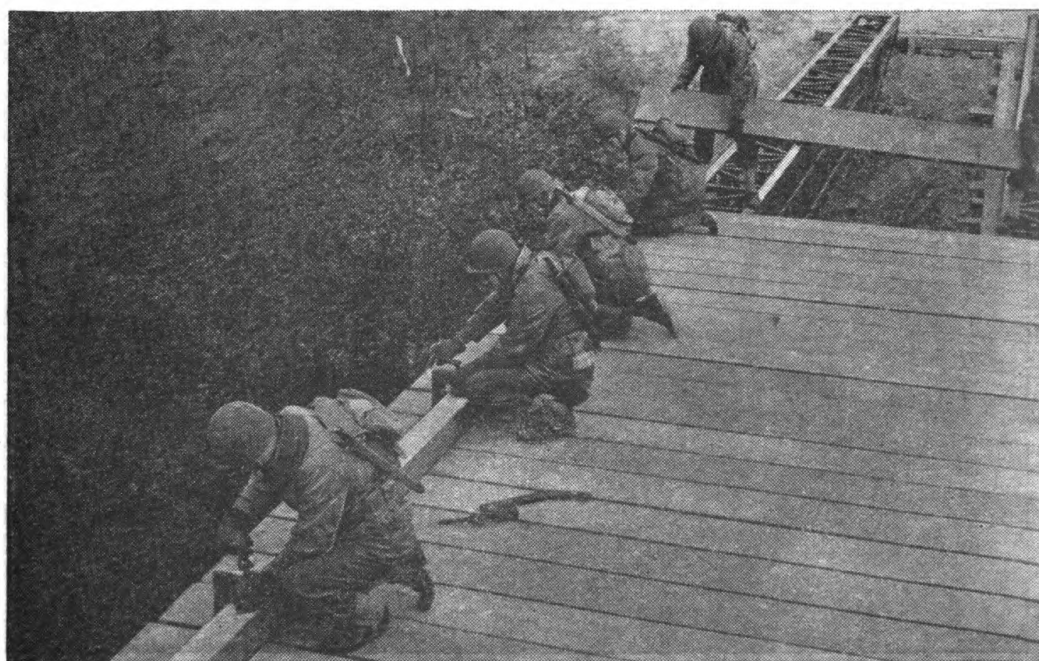
FIGURE 41.—Attaching siderails.
