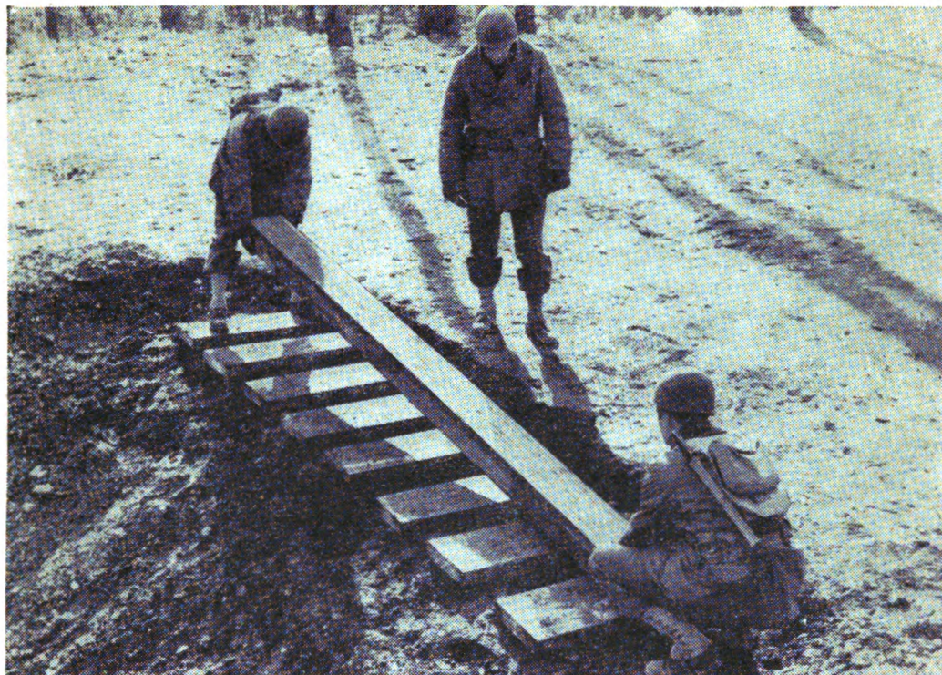
FIGURE 26.—Placing abutment sill on footings.
