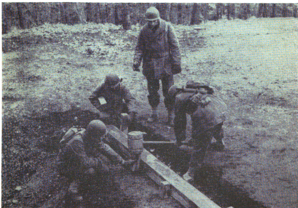
FIGURE 27.—Abutment sill being secured in place.
