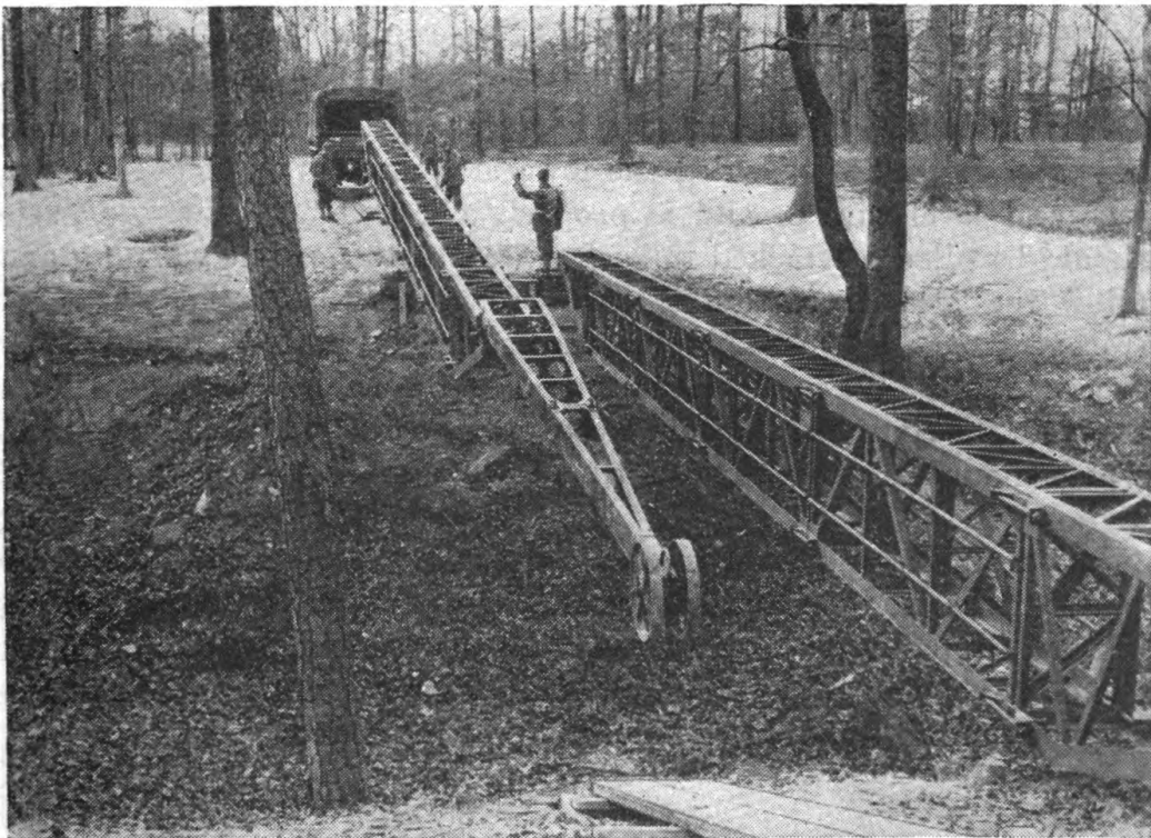
FIGURE 45.—Truss being hauled out by truck.
