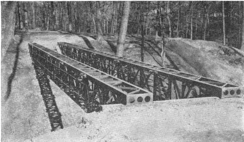
FIGURE 3.—Trusses in place across gap.
