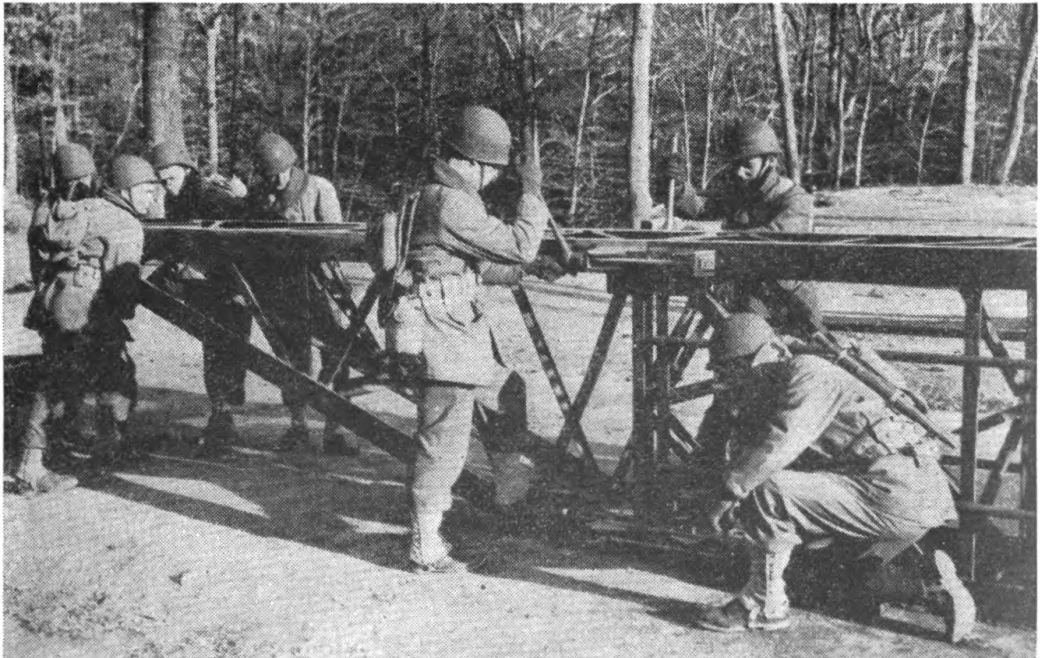
FIGURE 19.—End and intermediate sections being bolted together.
