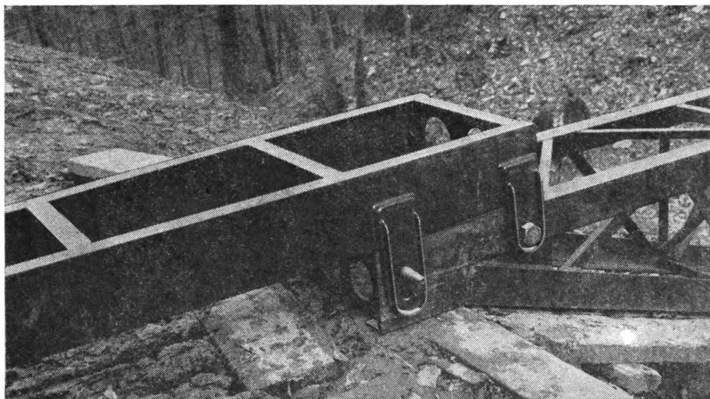
FIGURE 36.—Truss resting in place on abutment sill.
