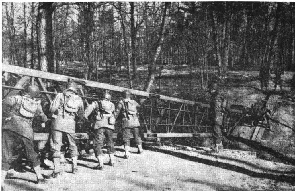
FIGURE 32.—Truss reaching far bank.
