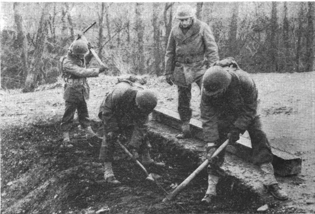
FIGURE 25.—Cutting down bank for abutment sill.
