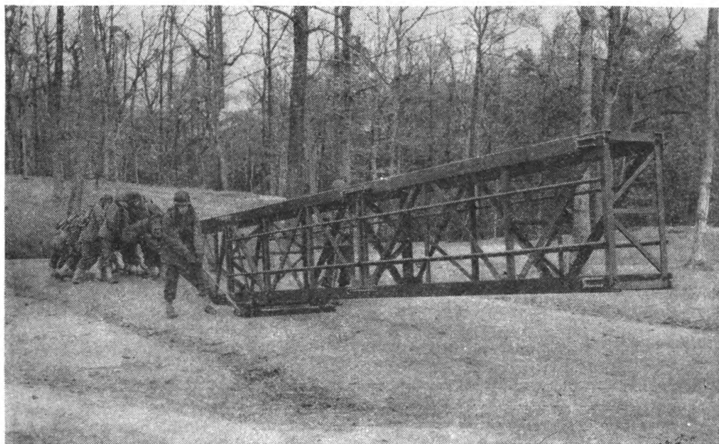
FIGURE 22.—Erection roller being inserted beneath truss.
