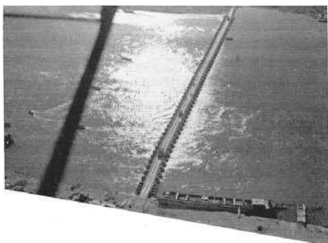
Vehicles cross Rhine on heavy pontoon bridge constructed by Corps Engineers at Kripp-Linz.
