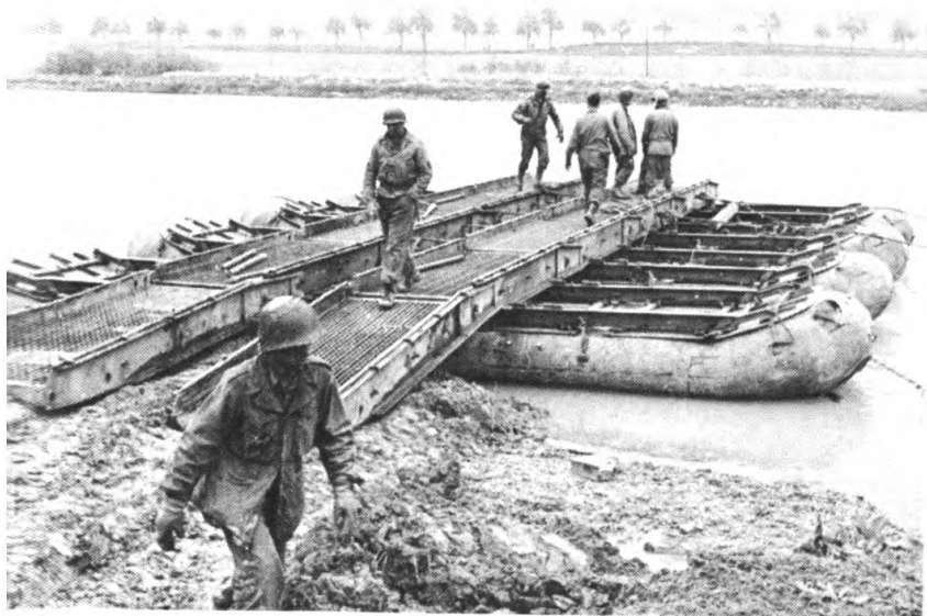
The bridge grows. Another section is hooked on.
