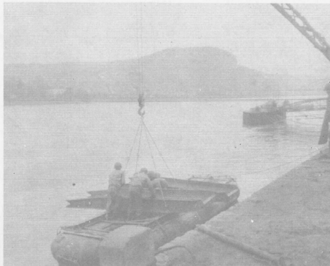
Construction of the Treadway Bridge.
